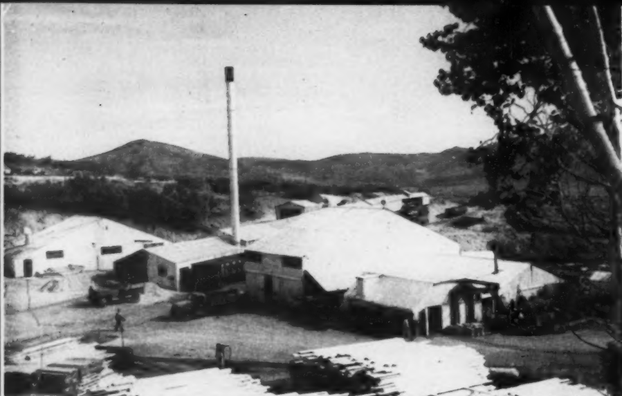
In this view of the Mayflower surface plant, the miners' change room is on the left; the steam plant near the center has a tall stack; the warehouse and shop is right of the steam plant, and the tipple is at the top center.
